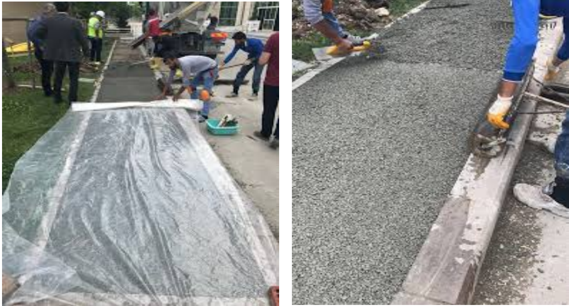
Figure 17: Ministry of Environment and Urbanisation Campus, Permeable Concrete Application 12
