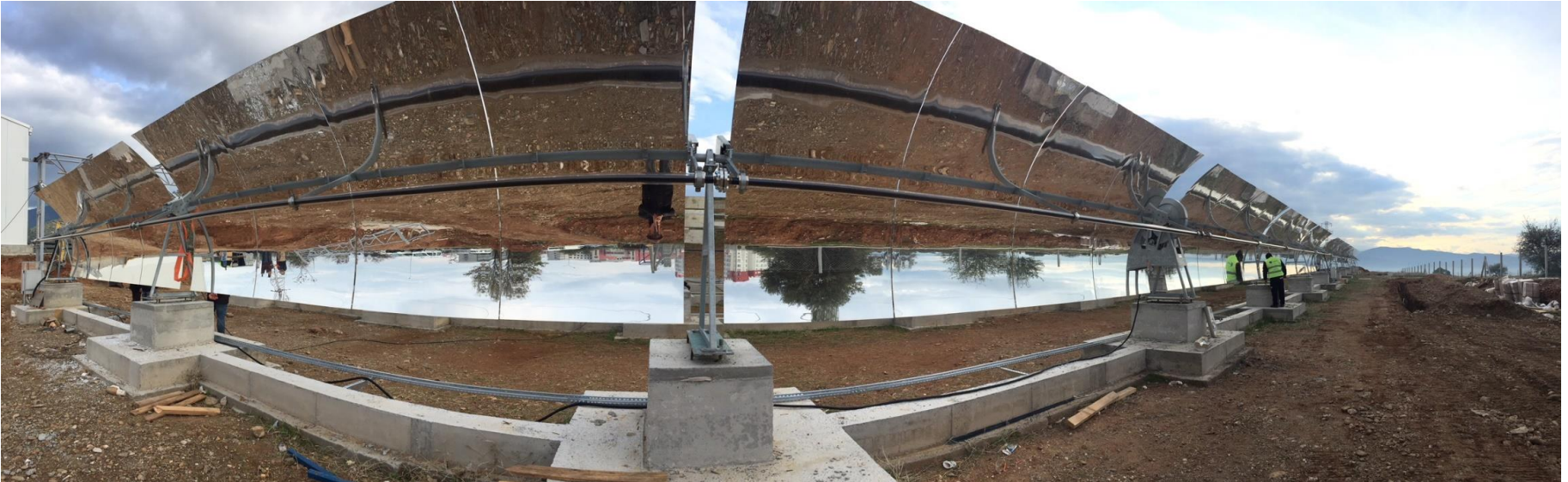
20 modules of the solar collector system PTMx-36 (SOL): Phase 1 Ground installation over separate foundations for each plate
